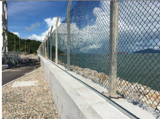
Cooling Water Intake for CCGT Unit No.1
