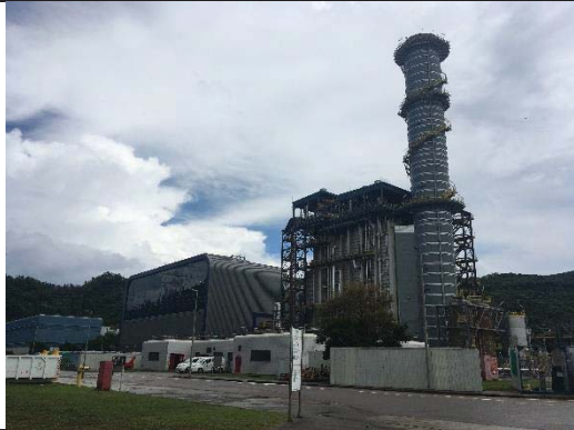
Generator Transformer and Turbine Hall of CCGT Unit No.1
