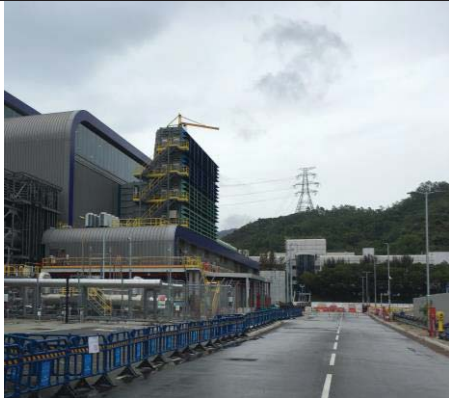
Reinstatement of road after the construction of CCGT Unit No.1
