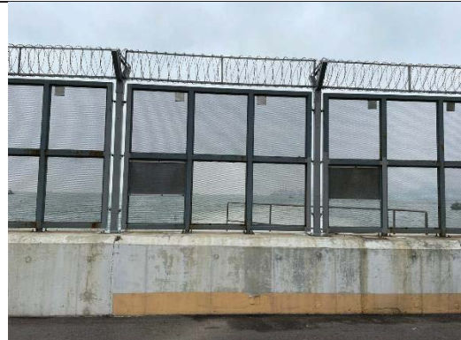
Cooling Water Discharge Facility for CCGT Unit No.1 and reinstatement of crest walls and fencing barrier
