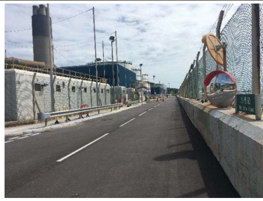
Reinstatement of road after the construction of Cooling Water Discharge Facility
